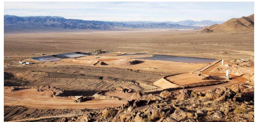
Overlooking Heap Leach & Process Facilities
